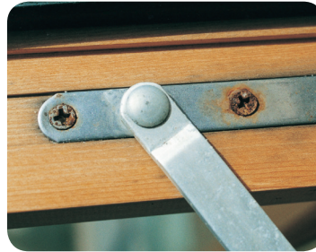
Screw holes when dissimilar materials are used.
